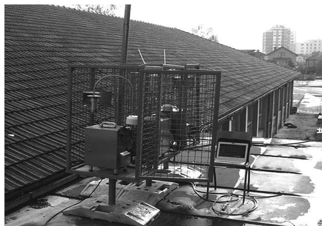
Fig. 2. The image for the outdoor air measuring instruments.
