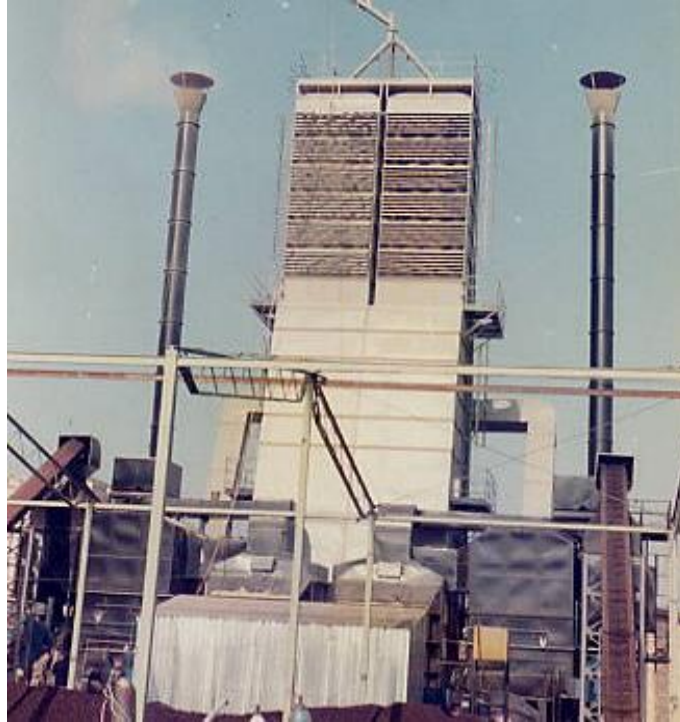
Vertical corn dryer, with 2x5MW FB furnace
